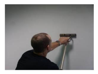
Trim the wall covering if necessary where it overlaps the flooring coved skirting taking care not to damage the floor covering. Roll overlaps and seams with a seam roller.
