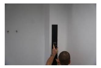
Apply adhesive right up to the horizontal line. See guidance above and the adhesive manufacturer's instructions for application, use and drying times.
